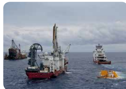
Vessels during buoy installation
